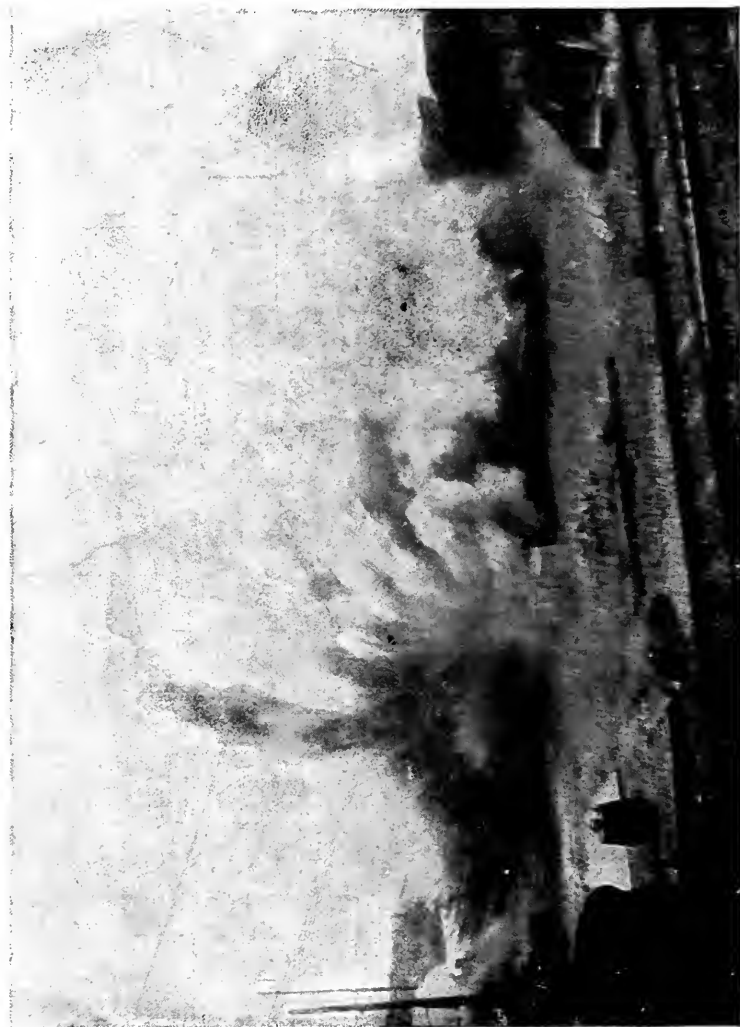
View at downcast end of large sheet of flame issuing from mouth of gallery to a distance of 180 ft. Length of coal dust zone 367 ft.
